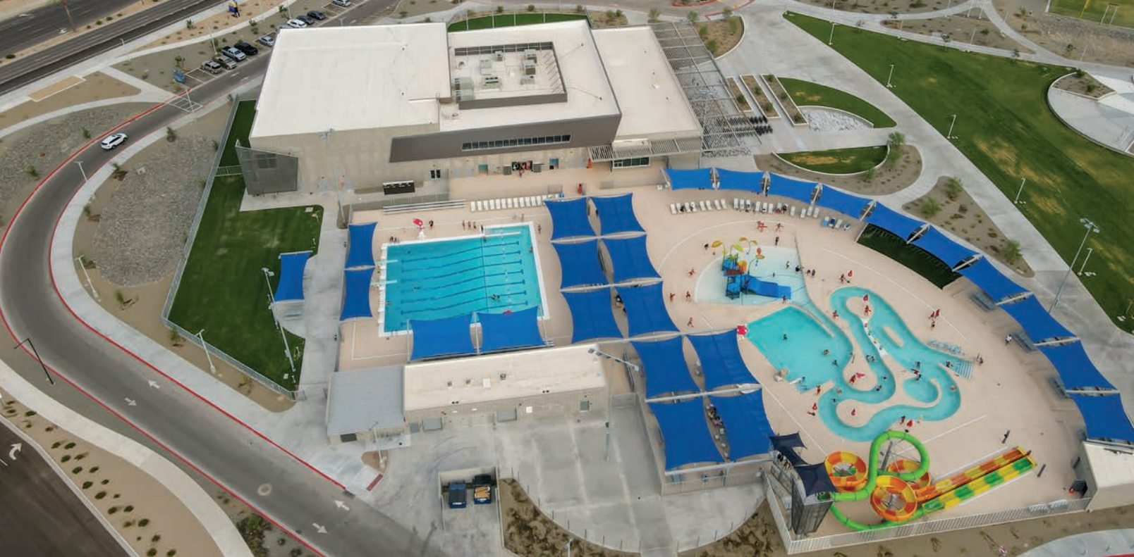
Above: Two acres of the allotted space was dedicated to the aquatics facility that includes a 25-yard, 8-lane competition pool, a leisure pool, a lazy river, a separate 27-foot-high dual slide tower along with a perimeter of shaded cabana areas.
