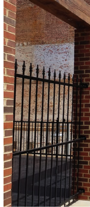
Above, Center: The park is accessed by a gate that gives way to a steel landing and opens up to both the stairs and a wheelchair lift. Custom iron fencing was constructed by local company, Reynolds & Easley Manufacturing. A repurposed beam above the gate provides continuity in streetscaping while adding visibility from the road.
