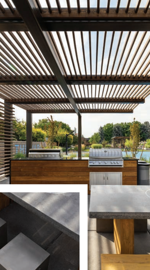
Above: Four concrete tabletops with wood legs work well with the shade structure and concrete patio. Each chair (inset) is a movable lightweight concrete block. The grill is 36" wide with a black granite countertop and tiger wood-stained cladded decking.
