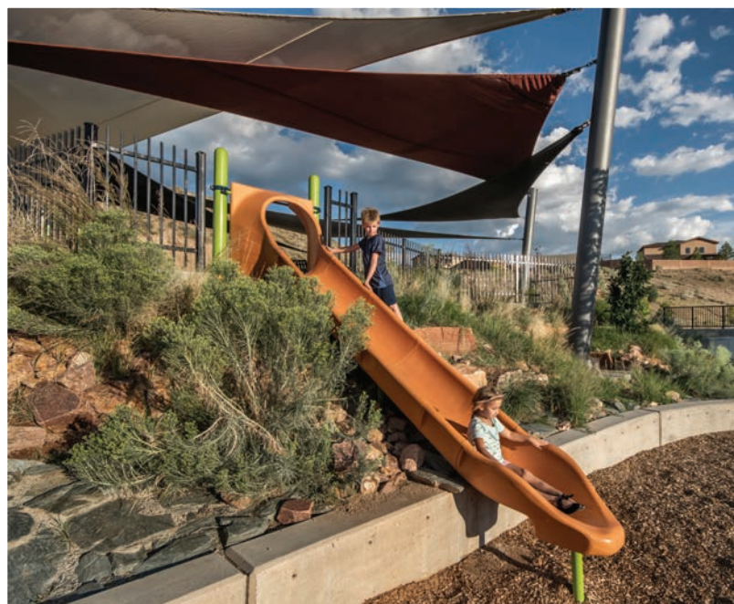
Right: The slide is composed of a molded plastic and leads to surfacing made of engineered wood fiber playground surfacing (EWF). That's the standard material MRWM uses in parks and schools in Albuquerque. It meets the safety guidelines for impact attenuation while also allowing lateral displacement if a child falls on it at an angle. It's also considered an accessible surfacing material.
