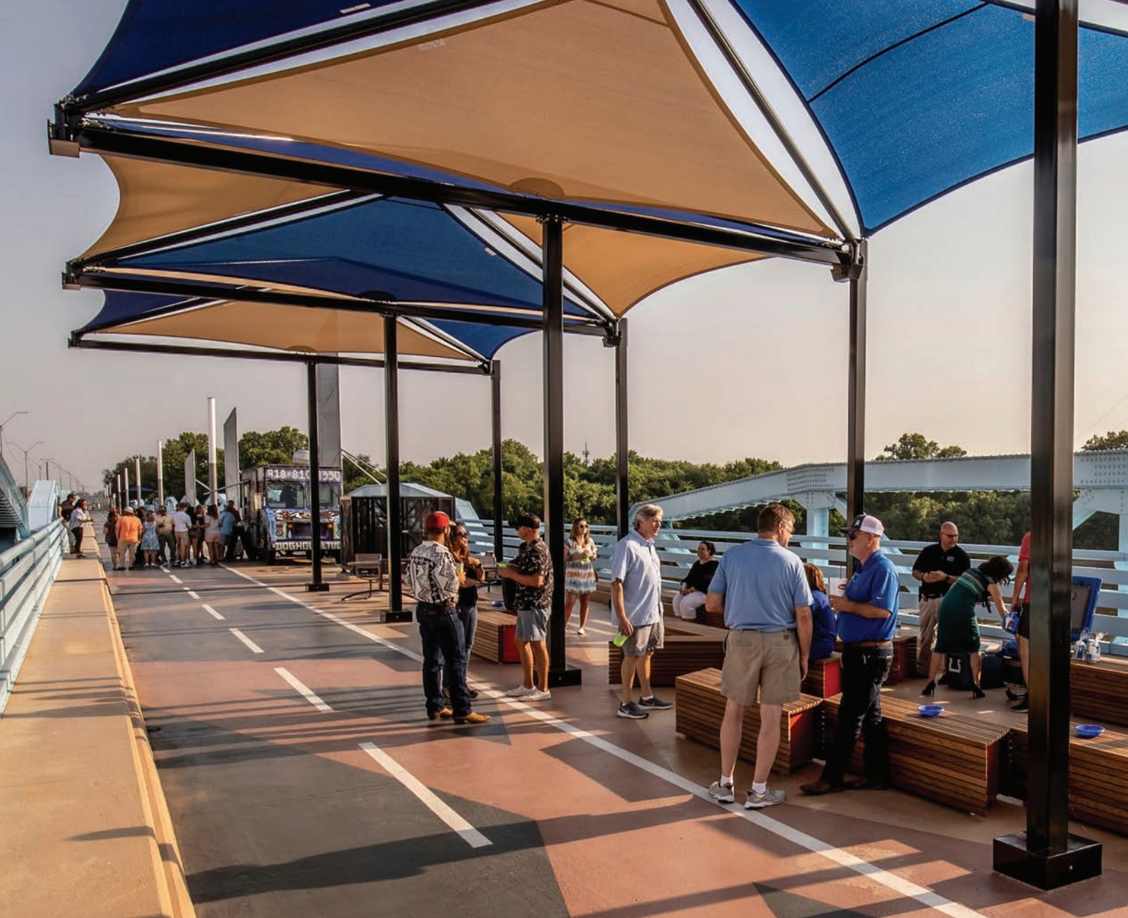
Above: The 2,000-linear-foot bridge can even house events with food trucks. The shade structures include a 25'x 100' custom cantilevered structure and 12' x 30' hip roofs. Underneath this shade structure are parallel benches made of lpe wood.
